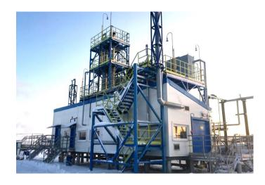
The modular design of the plant allows it to be assembled in the field as quickly as possible, modifications can be made to tailor the serial solution to the customer's conditions. The unit can be designed for harsh environmental conditions of the Far North.
